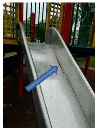
Fail - Separation between bedway and sidewall (see also below)
